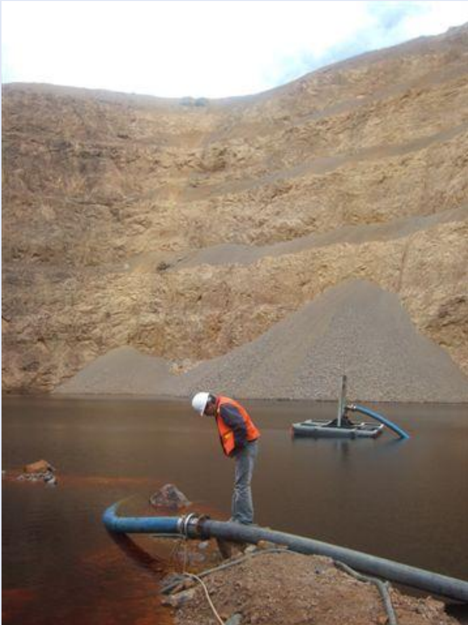
Dewatering collection pits
